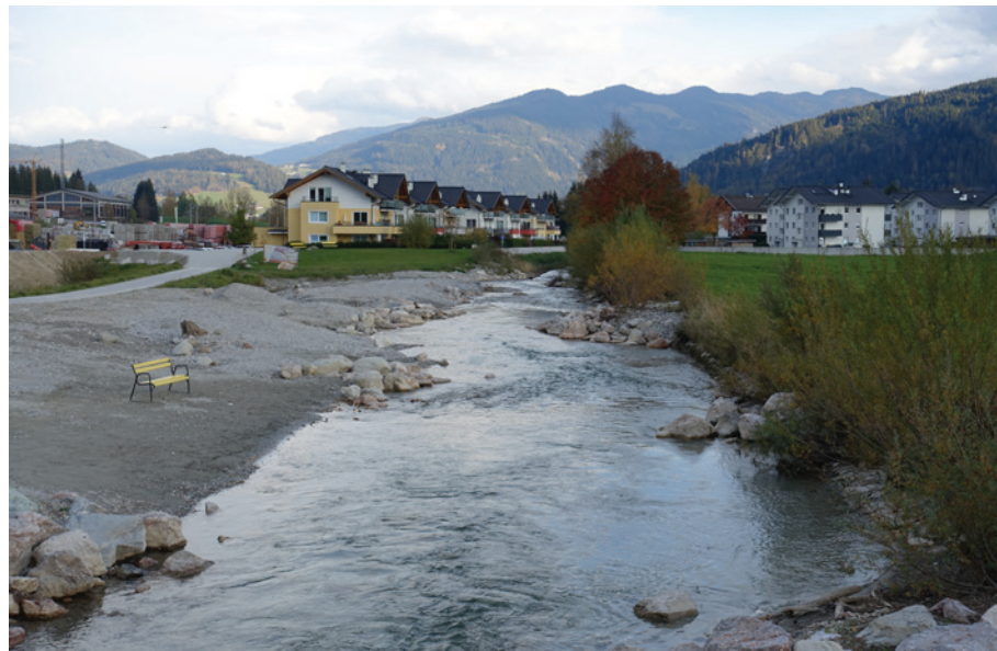
River widening in Altenmarkt (Austria)
