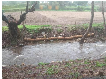
Figure 8. Biorolls used to retain sediments and/or riverbank stabilization.
