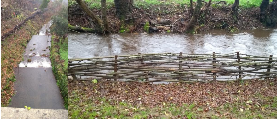
Figure 7. Live fascine NBS for riverbank protection.
