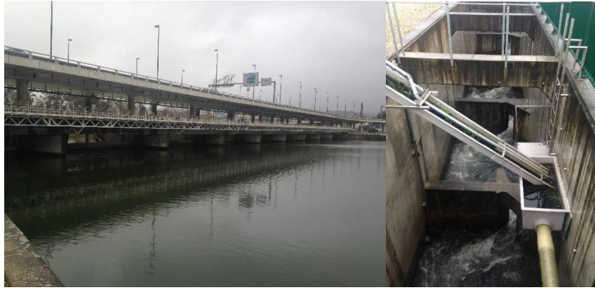
Figure 3. Açude dam in Mondego river(a), nearby Coimbra city centre, and associated fish passage (b).
