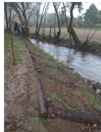
Figure 6. Living grade installed for riverine rehabilitation.
