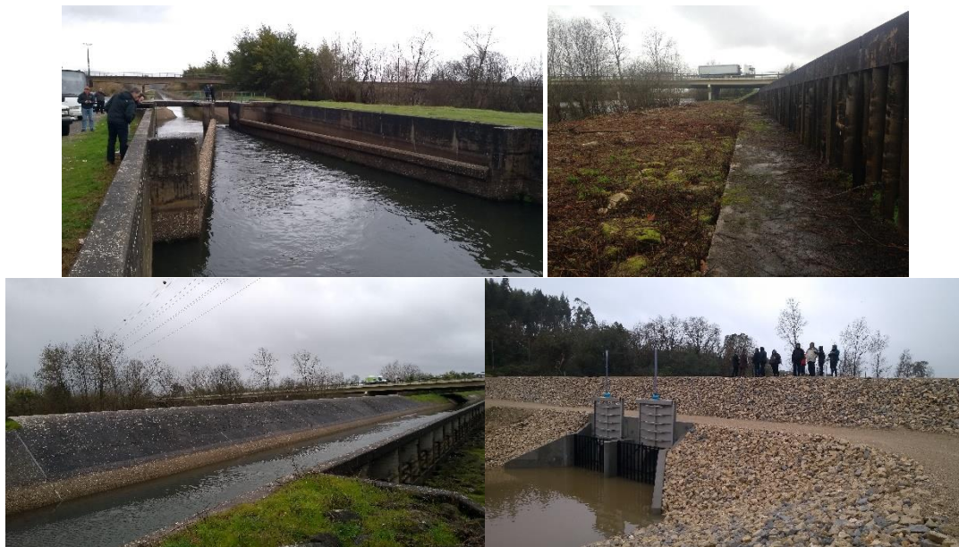
Figure 4. Hydraulic infrastructures used for water management in Mondego river: (a) flow monitoring, (b) area of supplementary water storage capacity (when flows increase from 1200 to 2000 m 3 /s), (c) secondary channel transporting water for irrigation of agriculture fields, (d) flood gates to protect lowland areas.
